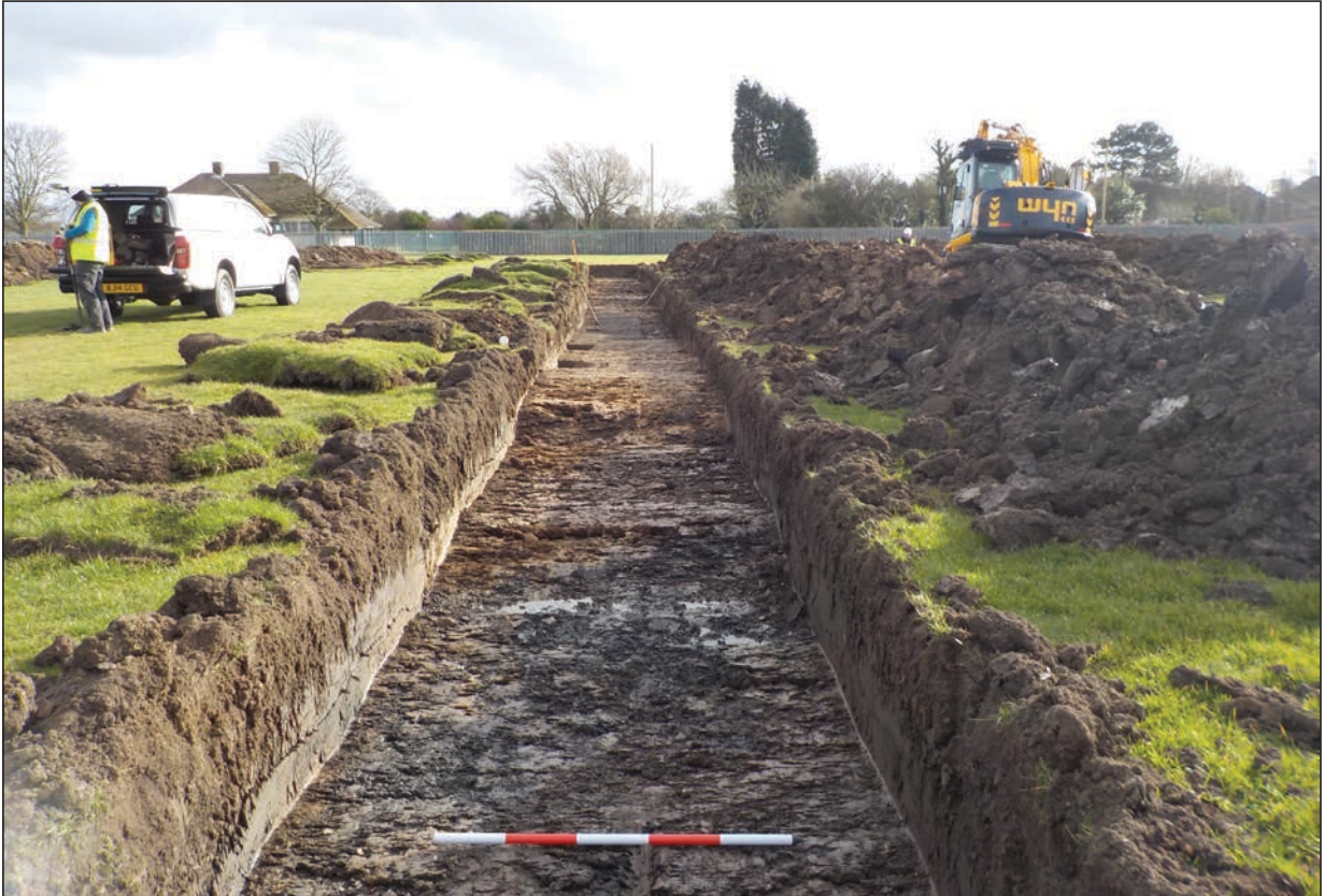
Plate 2 - View of Trench 2, facing SSE
