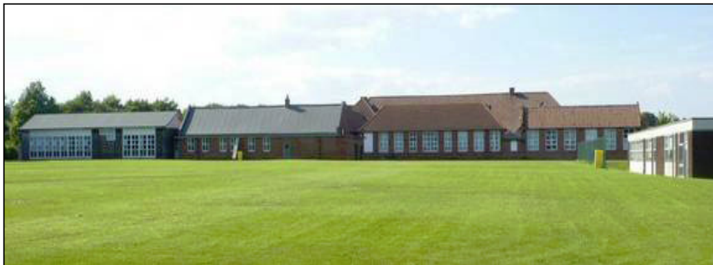
Plate 1 View of evaluation area prior to excavation
