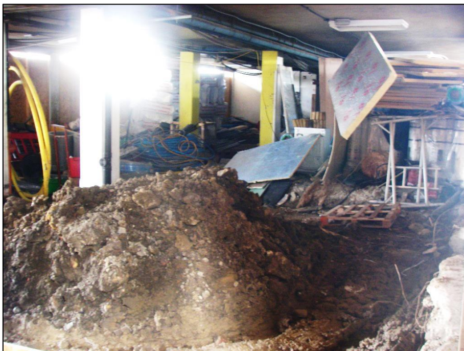
Photo 2: The view of the construction works beneath the present building
