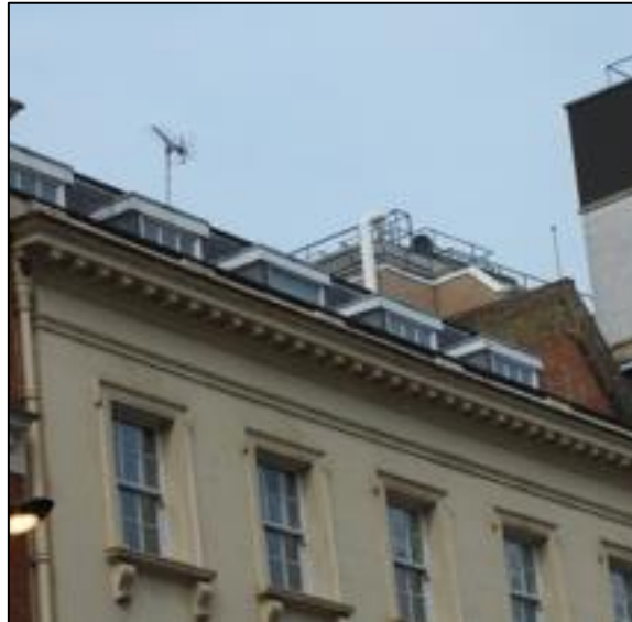
Photo 4: Yellow brick and metal railings marking the top of 22-23 Hanover Square
