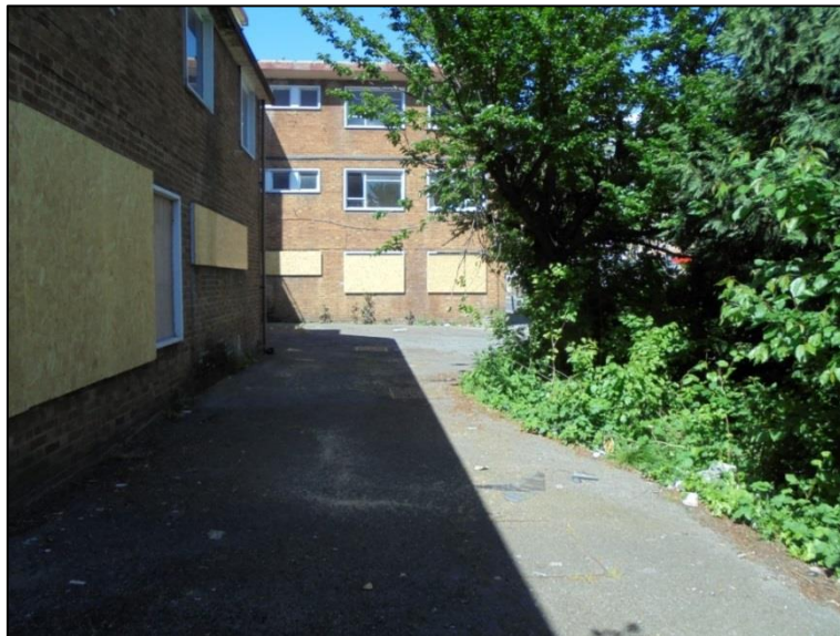
Photo 2: The view to the west from the building entrance on Southwark Park Road
