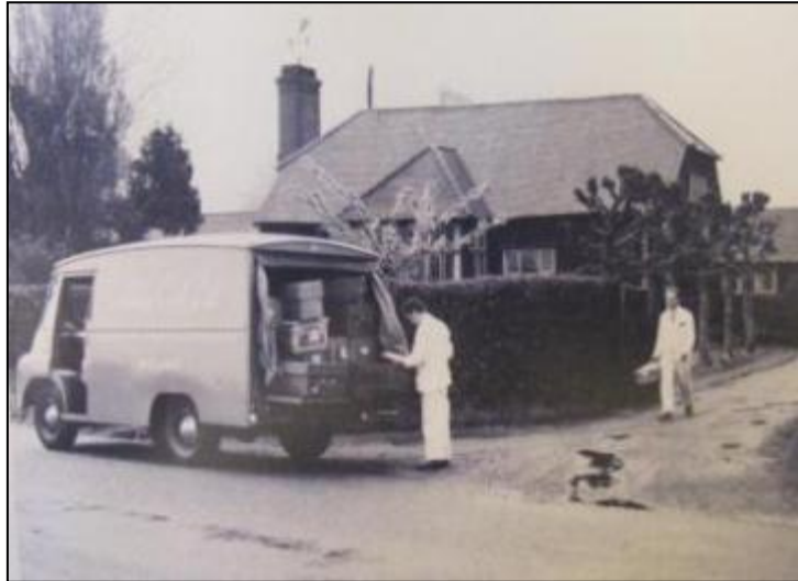
Plate 6: Part of the laundry buildings c. 1950's (z/540/13).
