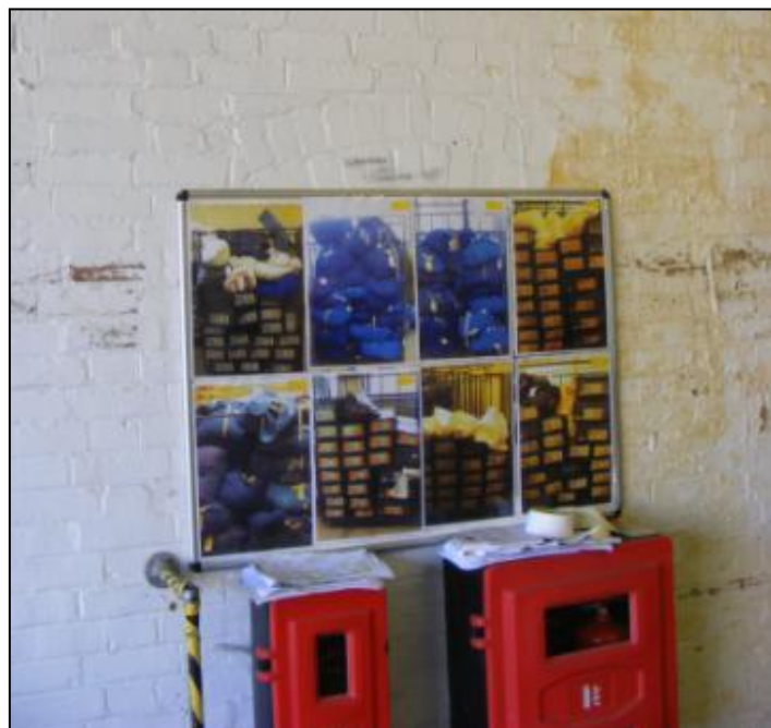
Photo 5: The curved segmented window arch is visible at the top of the notice board.
