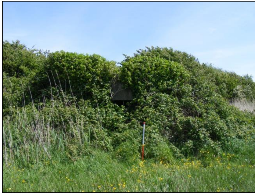
Photo 5: A pillbox [AB 11] at the north-eastern edge of section 1 within the proposed development site
