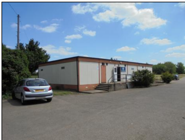
Photo 1: View of the car park and clubhouse from the north-west
