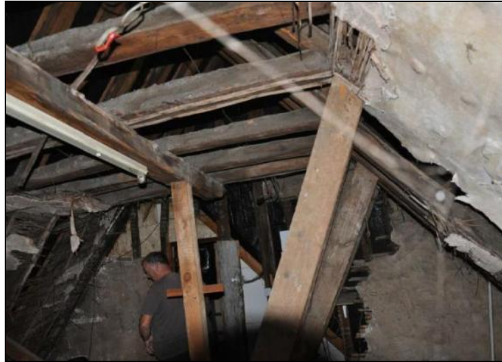
Photo 10: The plastered wooden lath stud walls and reed ceiling within the former attic space, taken during the early stages of the conservation works
