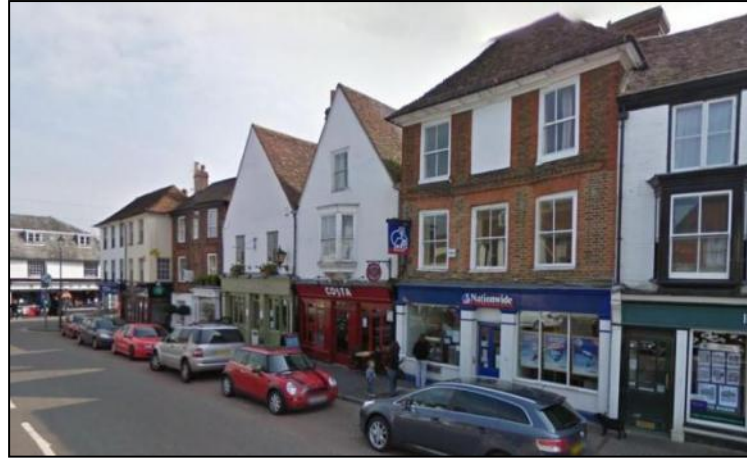
Photo 2: No. 65 High Street along the West Malling High Street. Viewed from the south-west prior to the refurbishment works
