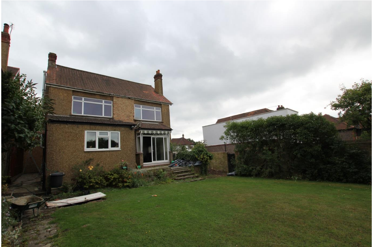
Plate 4: Rear elevation, showing relationship with 30 Ryecroft Road
