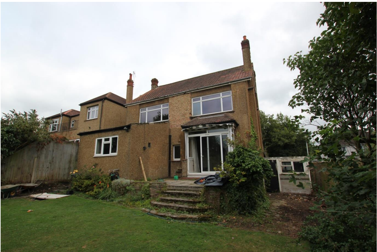
Plate 3: Rear elevation, showing relationship with 26 Ryecroft Road
