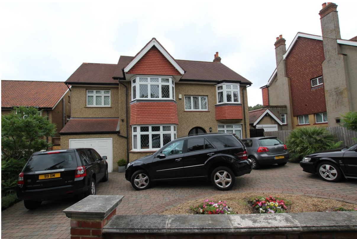
Plate 14: Part of the same row along Ryecroft Road, which makes a positive contribution
