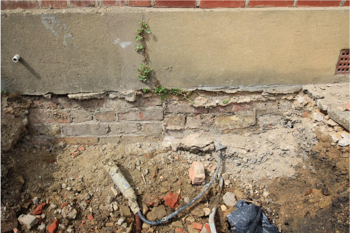
Plate 6: Phased brickwork on front elevation (right of the door)
