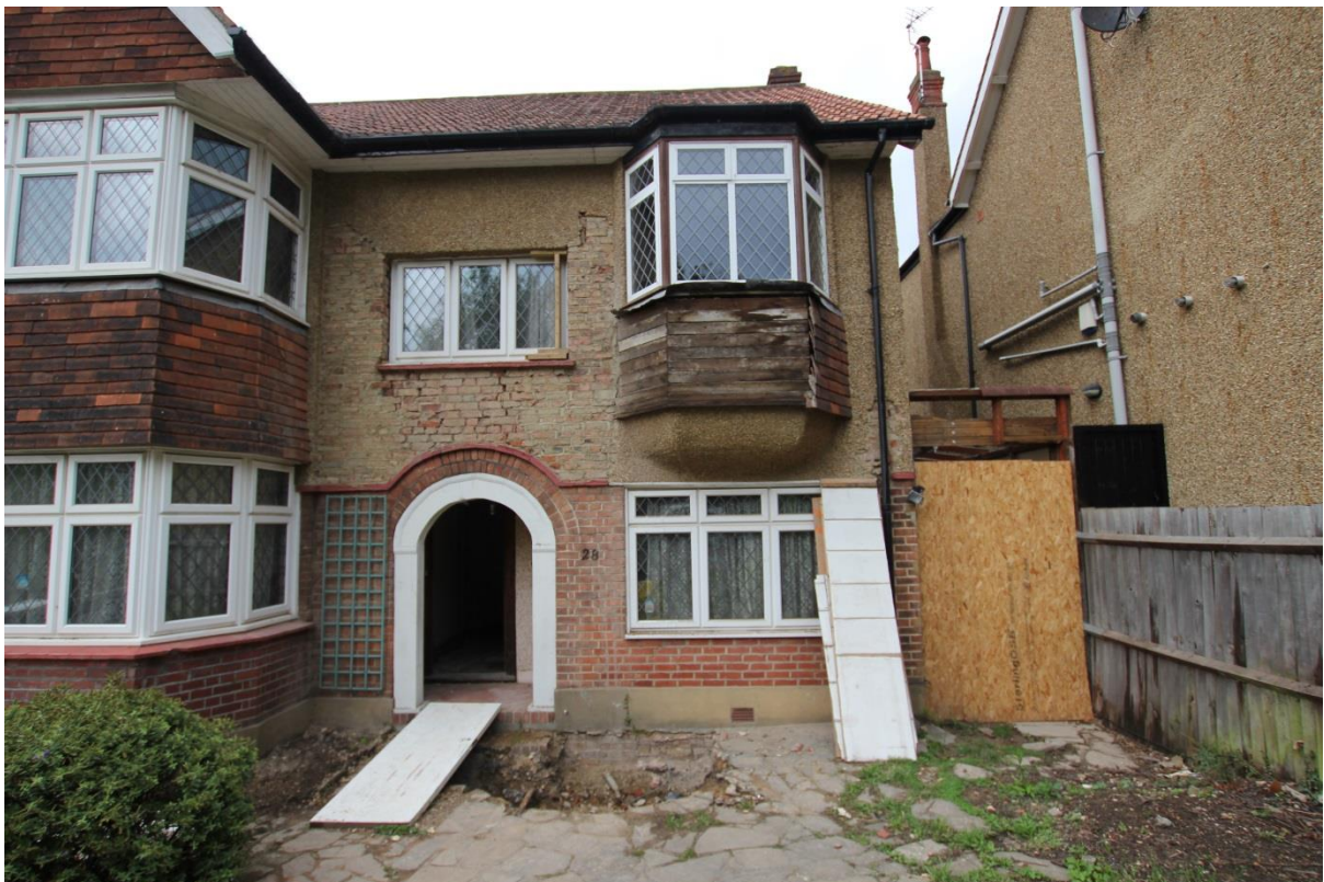
Plate 5: Front elevation, showing exposed brickwork and later alterations (probable replaced garage)
