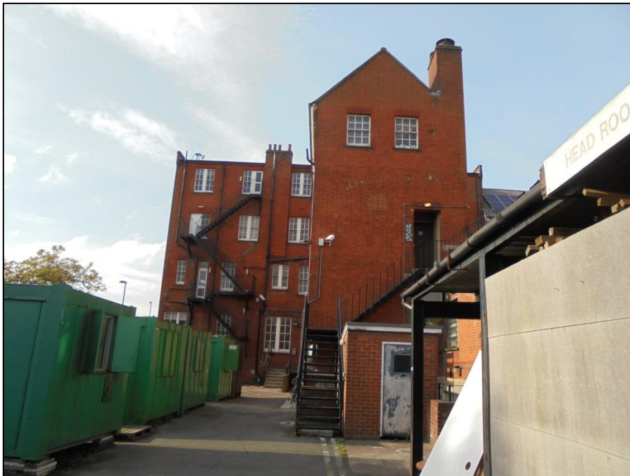
Photo 2: The rear of the building from the eastern site boundary
