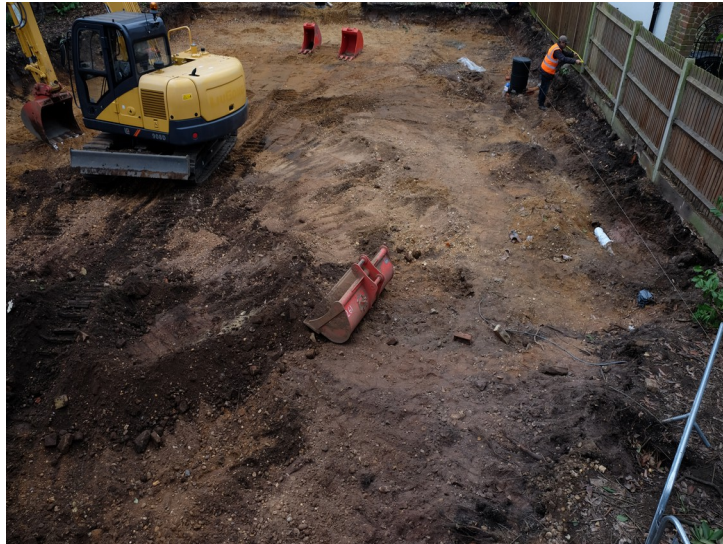
Plate 3 - Disturbed North Area of site. Facing West.
