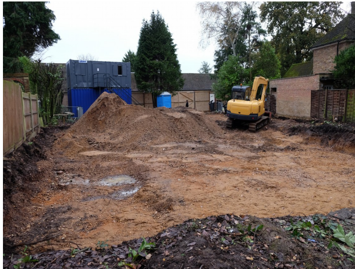
Plate 2 - Site stripped to natural. Facing East.
