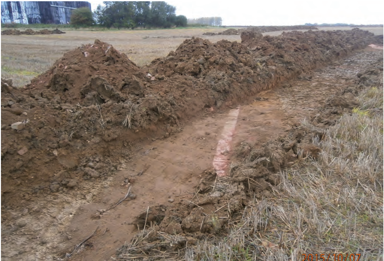
Plate 18 - Trench 3.05, firing-range wall [3017], facing northwest
