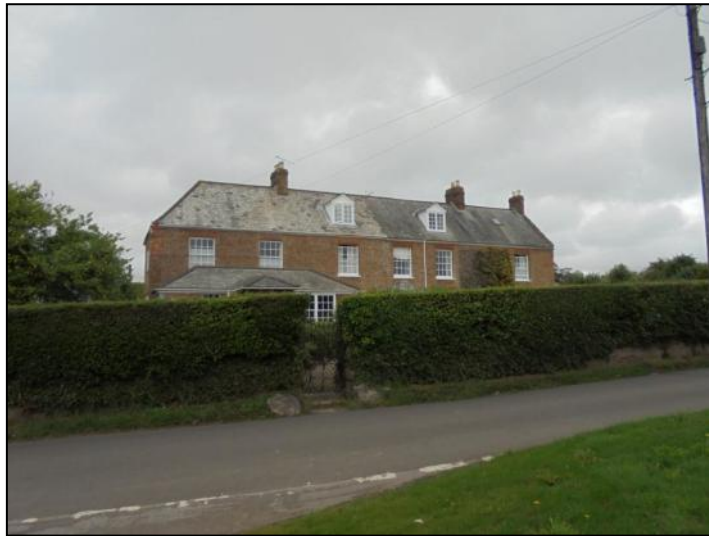
Photo 8: View of the front of Pyrland Farmhouse [AB 4] from the south
