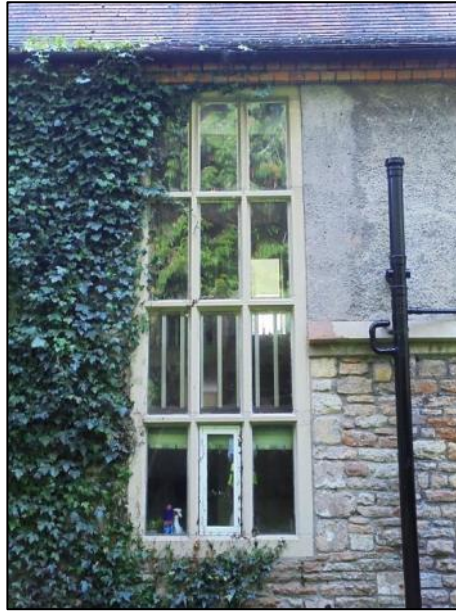
Photo 4: Mullion window on northern elevation, from the north
