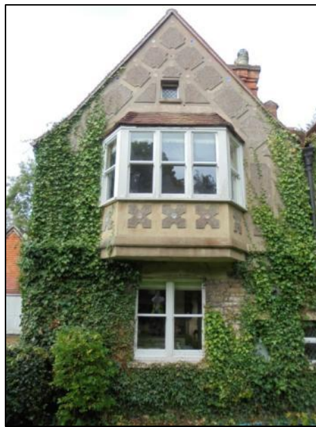
Photo 3: Southern gable of eastern elevation, from the east
