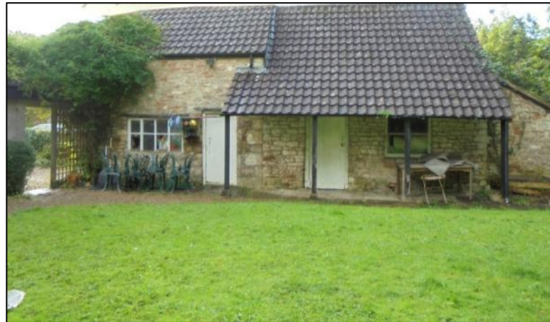
Photo 7: Eastern elevation of the outbuilding, from the north
