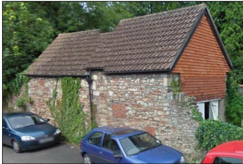
Photo 5: South elevation of the outbuilding, from the south-east (online source)
