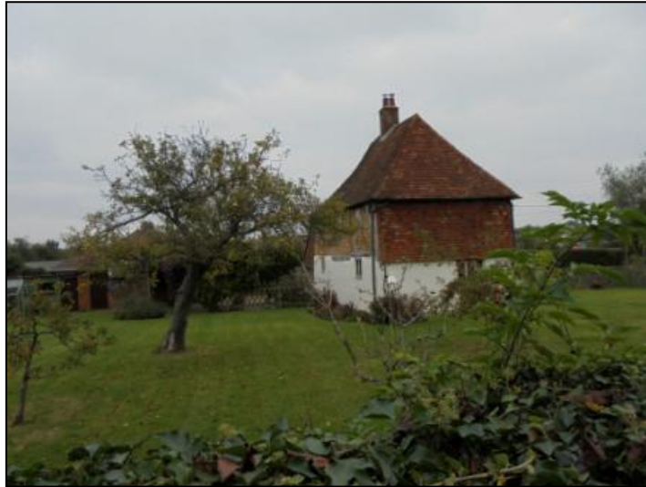
Photo 8: Ye Old Cottage [AB 16], from the south-west
