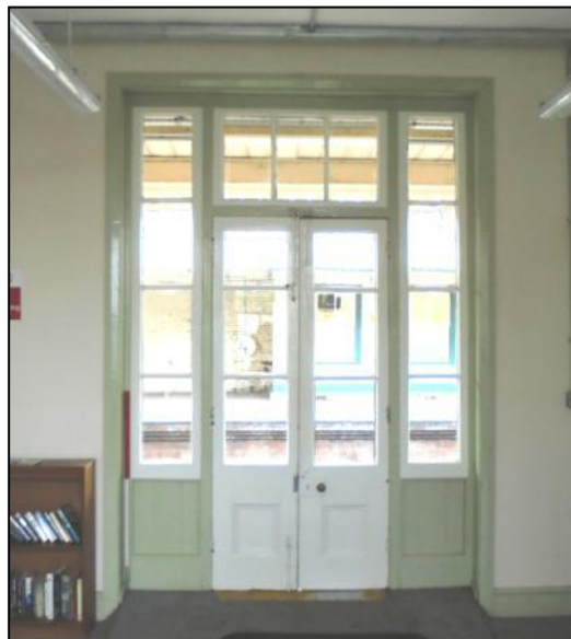
Photo 6: Interior of the waiting room door from the south, scale 1m
