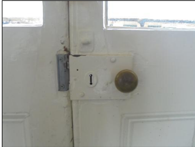
Photo 7: Mortice lock, brass knob and hook plate on the interior of the waiting room door
