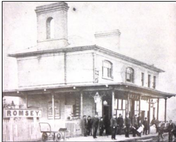
Plate 1: Romsey station in c. 1884 from the north-east (Cousins, 1983)
