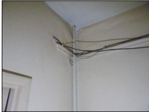
Photo 8: Picture rail turning a corner, now within a hallway outside room 3 on the first floor
