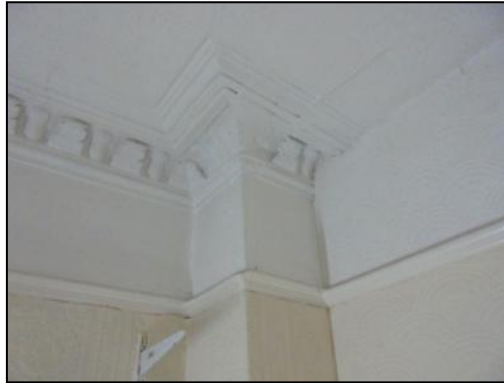
Photo 7: Truncated coving and picture rail in room 1 on the first floor
