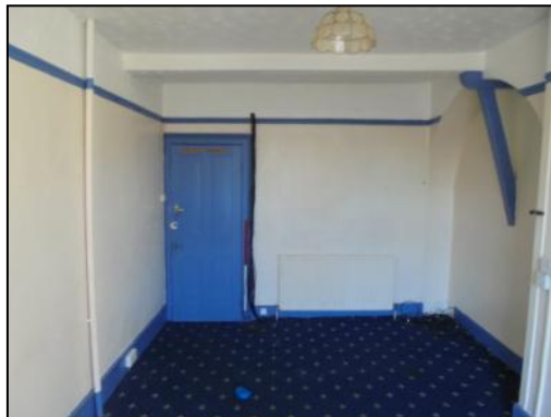
Photo 9: Alcove and beam within room 4 on the first floor, scale 1m
