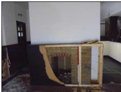
Photo 5: Main chimney on the Ground floor, scale 1m
