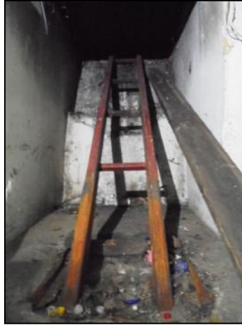
Photo 4: Rails in the basement floor
