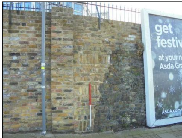
Photo 3: Adjoining sections of wall at the north-east corner, scale 1m
