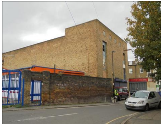
Photo 4: View of the warehouse building from the south-east
