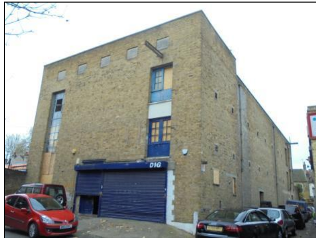
Photo 2: East elevation of the warehouse building, viewed from the north-east
