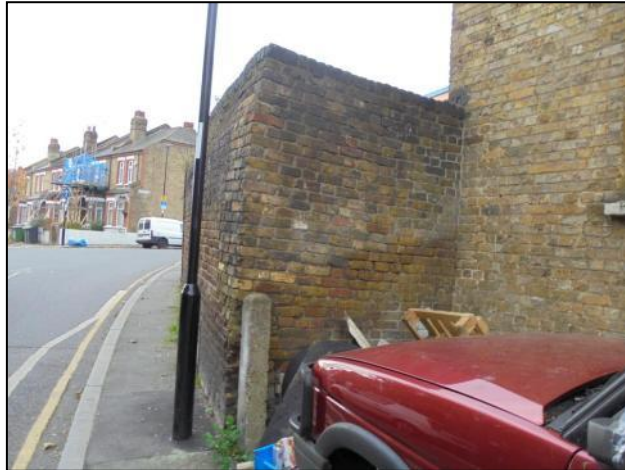
Photo 8: Boundary wall abutting the warehouse building, viewed from the north-east
