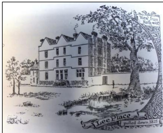
Plate 1: Lee Place, viewed from the north-west (Gregory et al , 1923)
