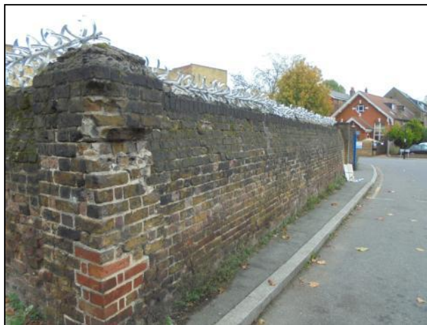
Photo 7: The boundary wall, viewed from south-west
