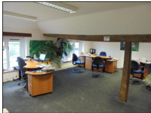
Photo 4: Tie beam, first floor of Building 2
