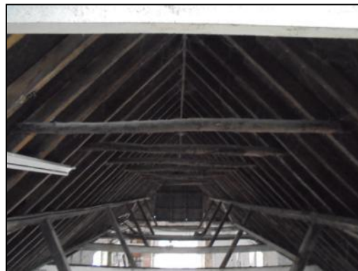
Photo 2: South-western roof section of Building 1
