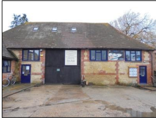
Photo 3: North-east elevation of Building 2 (scale 1m)
