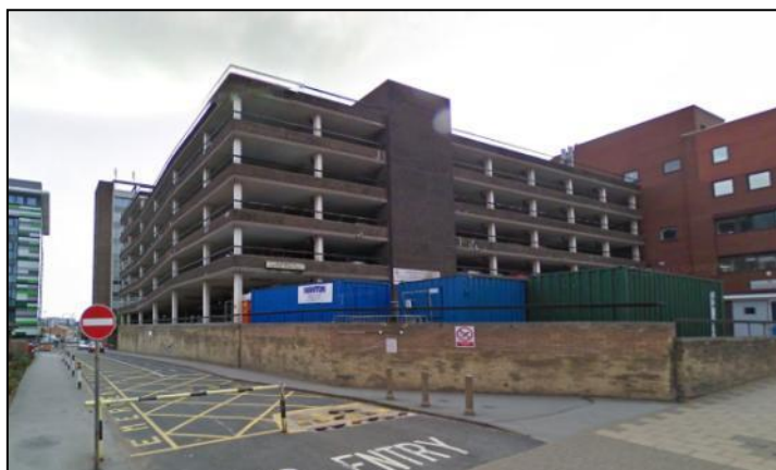
Photo 1: The former multi-storey car park in 2011 (Google Street View)
