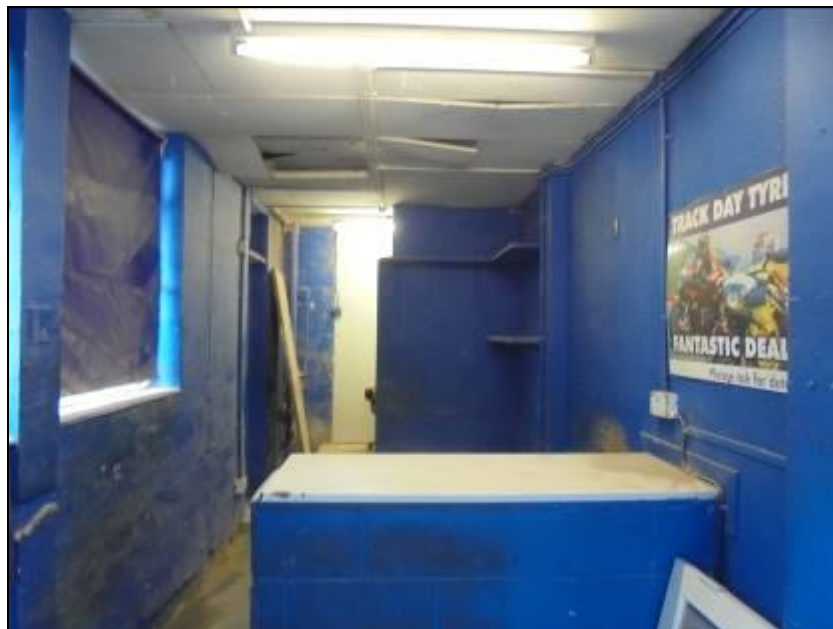
Photo 2: The southern room within the brick structure in the north-east of the site, taken from the south looking north
