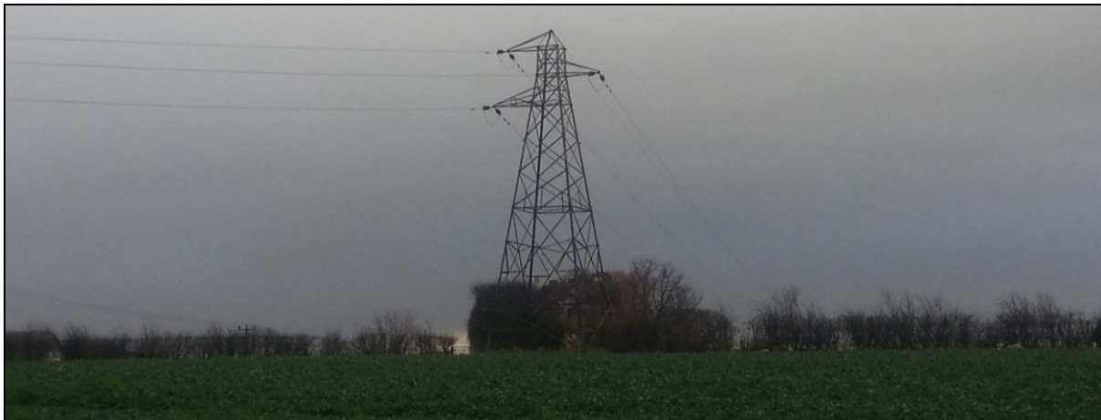
Plate 2 Electricity Pylon taken from the north of the site facing south
