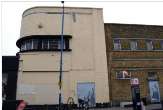
Photo 2: South-west corner of No. 89-93 (Scale 1m)
