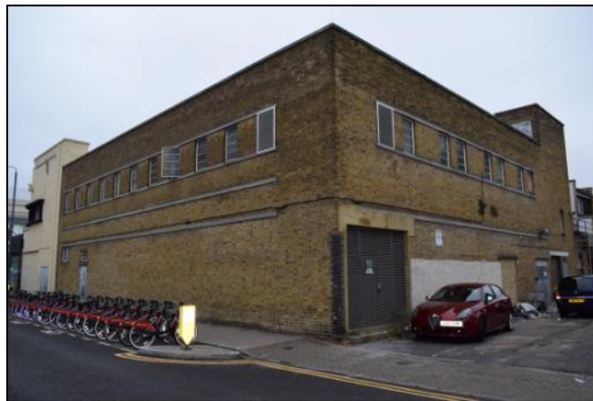
Photo 5: Southern and eastern elevations
