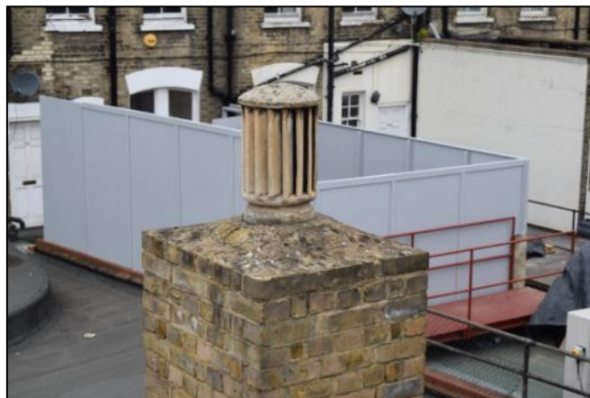
Photo 10: 1930s chimney pot
