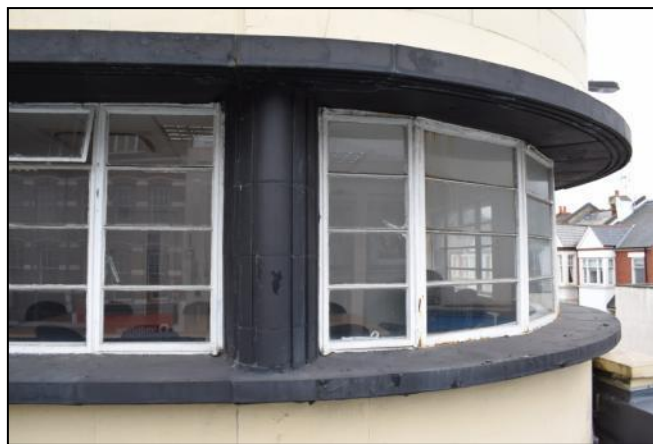
Photo 3: Sun trap window at south-west corner
