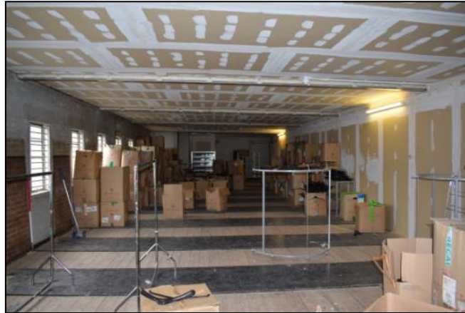
Photo 9: Original stock room on the first floor with polished concrete floor bays and original paint scheme (far left). Scale 1m.
