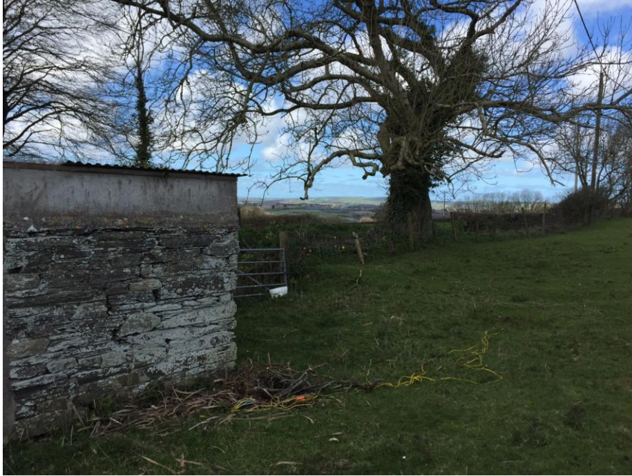
Plate 3: Building in SW corner of site, looking north-west.
