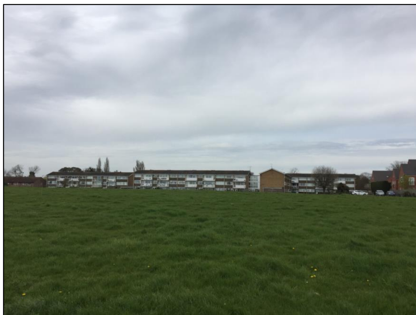
Plate 2: View of northern boundary, facing north
