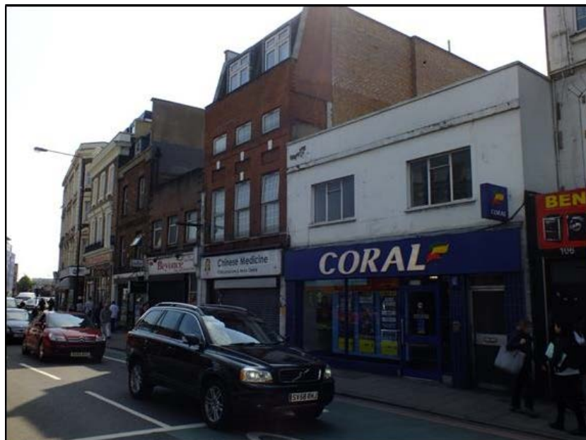
Photo 4: Northern façade and adjacent properties looking south-east
