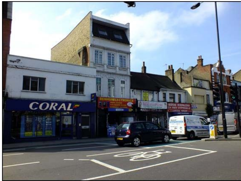
Photo 5: Northern façade and adjacent properties looking south-west
