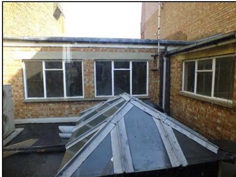
Photo 2: Central roof and skylight from 1st floor back room looking north
