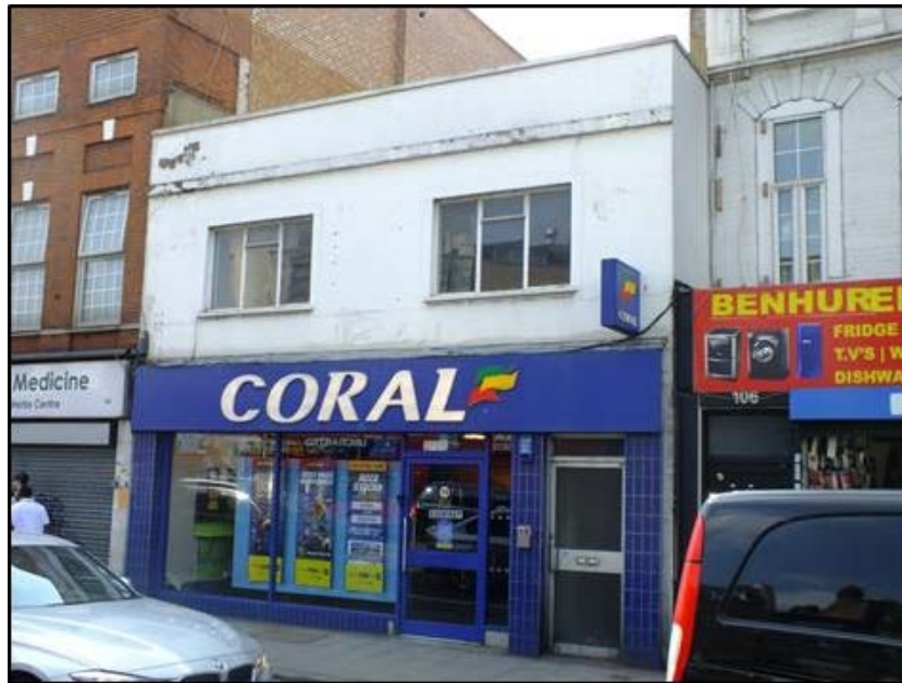
Photo 1: Northern façade from Peckham High Street looking south-east
