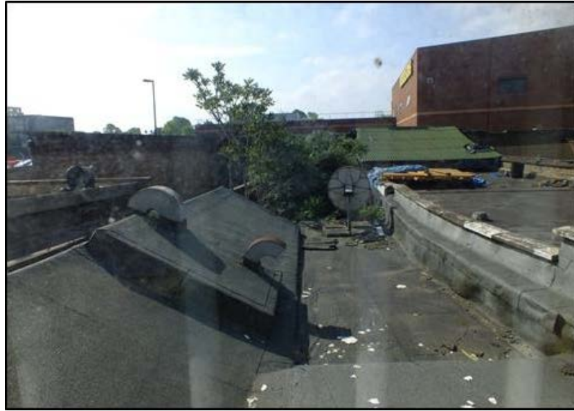
Photo 3: Rear of property from 1st floor window looking south-east
