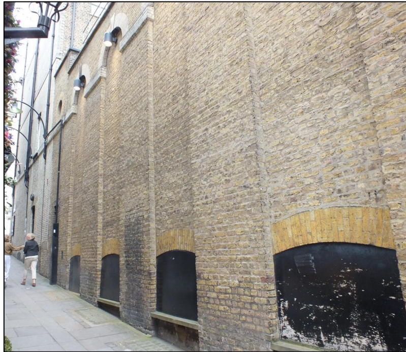
Plate 12: Northern façade, showing ground sloping, looking east
