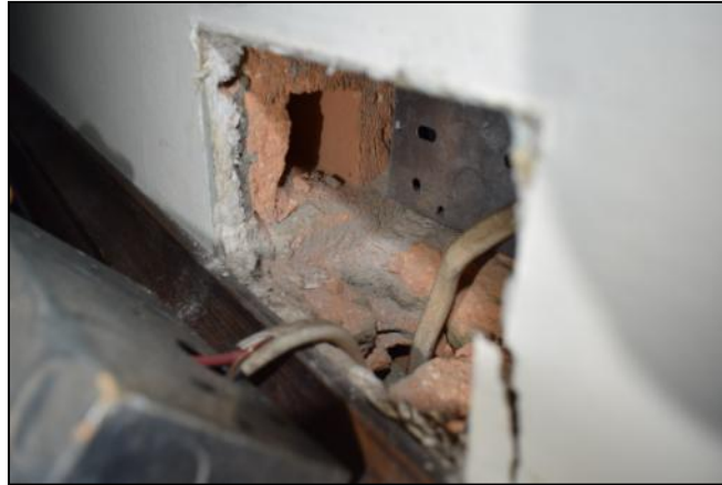
Photo 7: Industrially produced bricks behind the electrical plug socket
