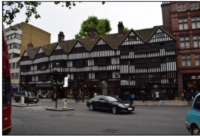
Photo 1: View of Staple Inn from Holborn (No. 4 is third floor, far left)
