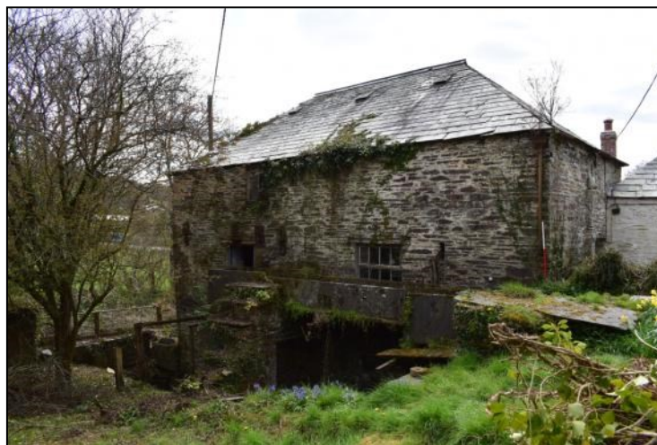
Photo 2: Eastern elevation of the mill with wheel pit & launder. Scale 1m
