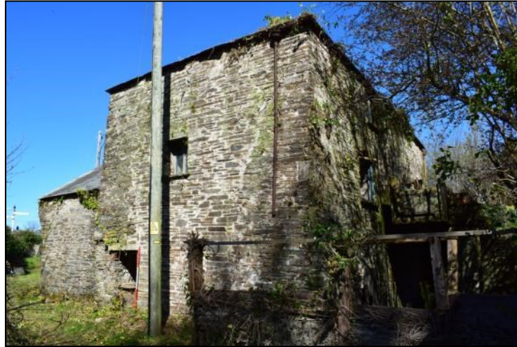
Photo 5: Southern elevation, Scale 2m
