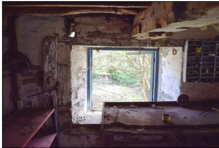
Photo 10: Launder sluice gate mechanism on the first floor
