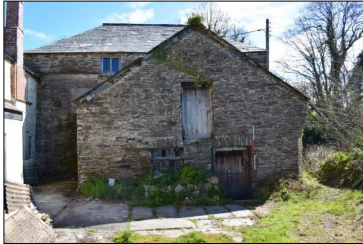
Photo 6: Western elevation, Scale 2m
