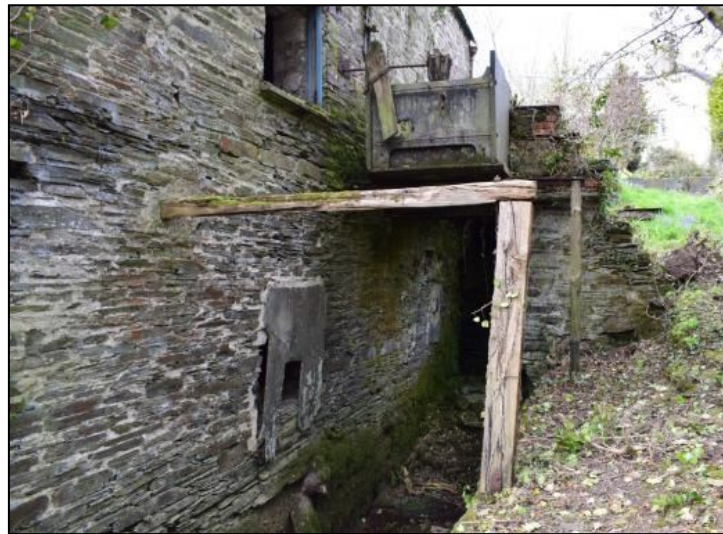
Photo 3: The wheel pit, launder and waterwheel apertures, from the south
