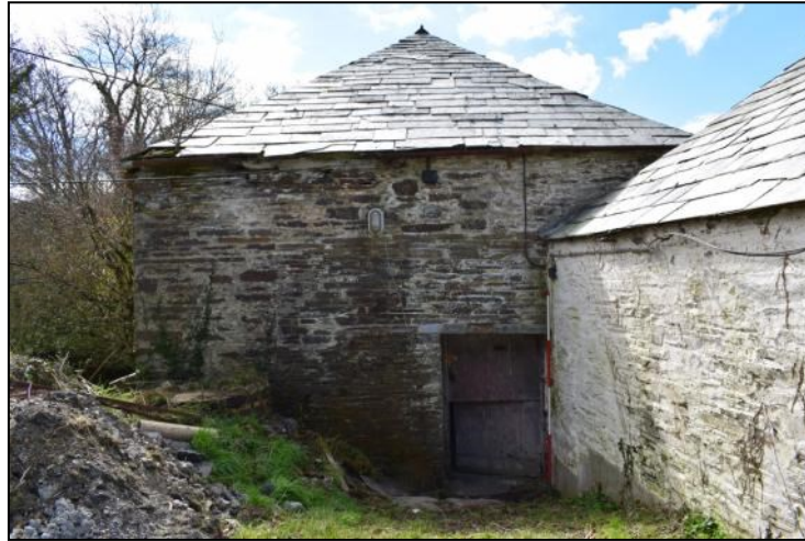
Photo 1: Northern elevation of the mill. Scale 2m
