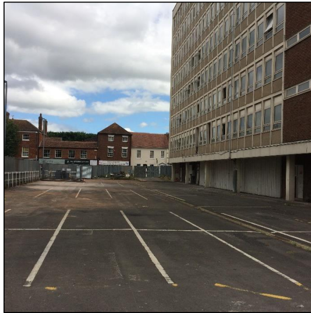
Photo 1: The northern facade of Quantock house, viewed from the west
