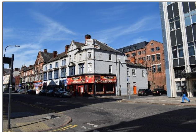
Photo 12: View from the corner of Humberstone Road and Morledge Street towards the site
