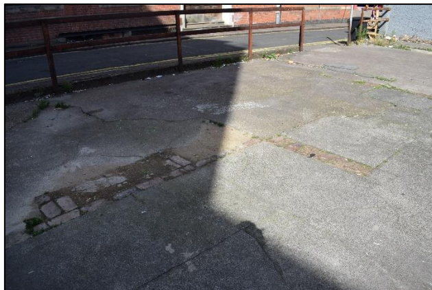
Photo 3: Brick foundations and possible floor within the site
