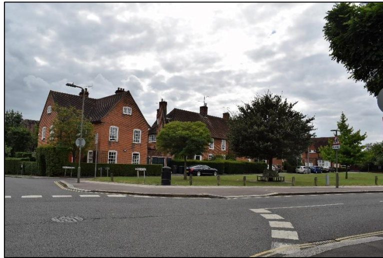
Photo 3: View of 115 Willifield from the corner of Asmunds Hill
