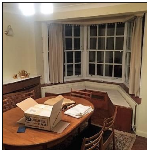
Photo 7: Secondary glazing at the dining room windows (February 2016)
