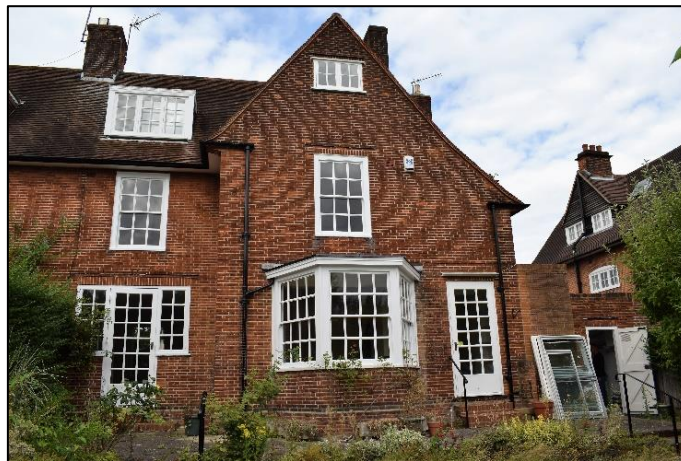
Photo 5: Rear elevation from the rear garden
