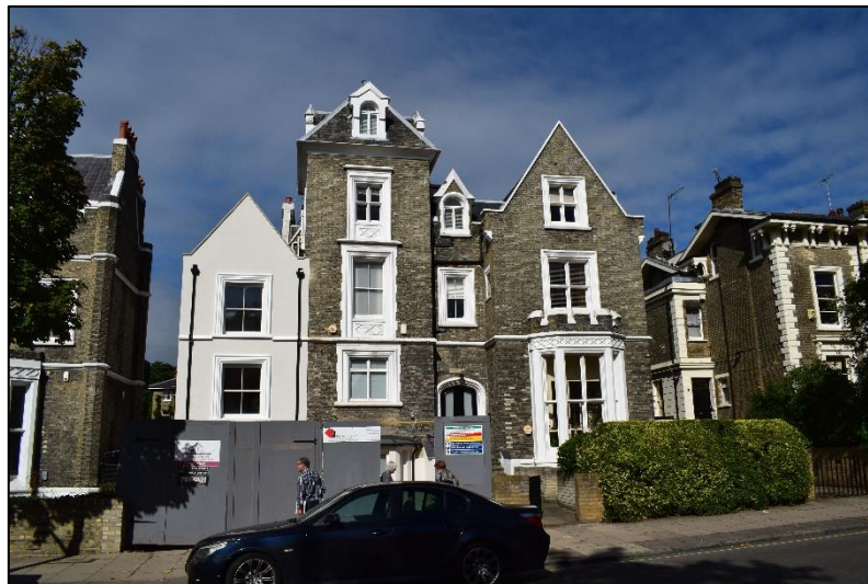
Photo 17: South elevation following redevelopment works
