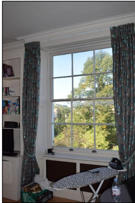
Photo 15: Panelled window reveal and cornice in first floor flat
