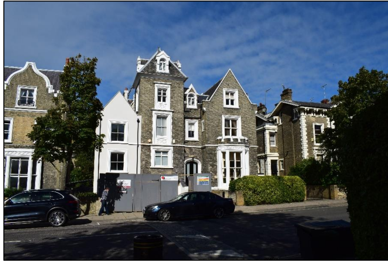
Photo 1: 84 Carlton Hill viewed in relation to the adjacent villas
