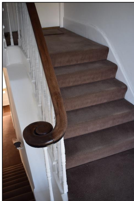
Photo 14: Elements of the original stairwell survive
