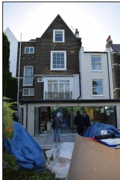
Photo 18: The north elevation following the redevelopment
