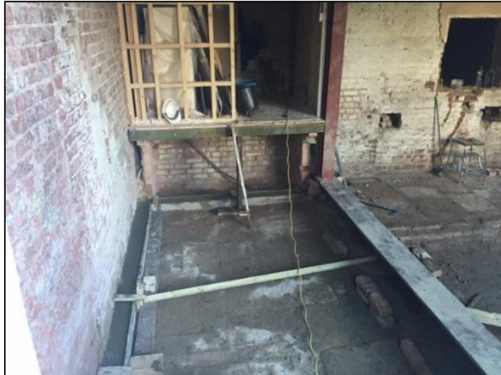
Photo 11: Stone floor slabs found during redevelopment works (Building Logistics Ltd)
