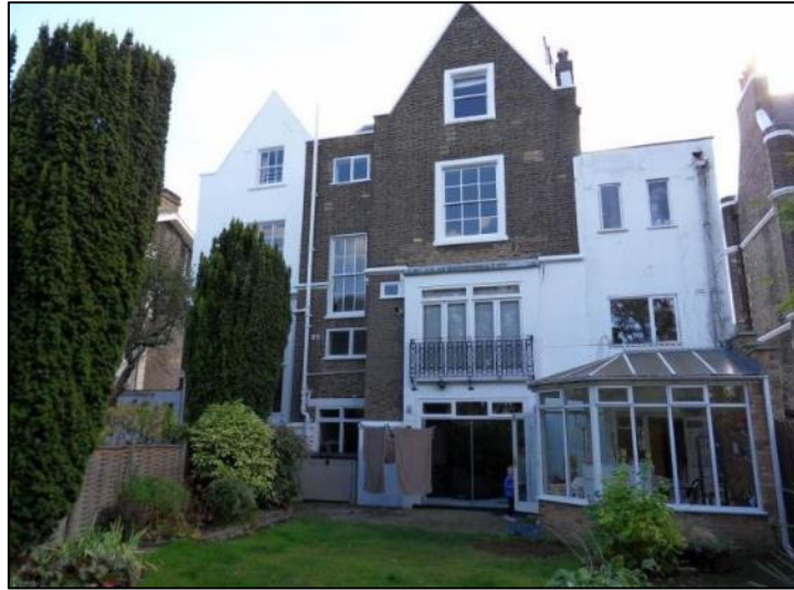
Photo 6: North elevation prior to the redevelopment (Gemini Building & Design Consultancy)
