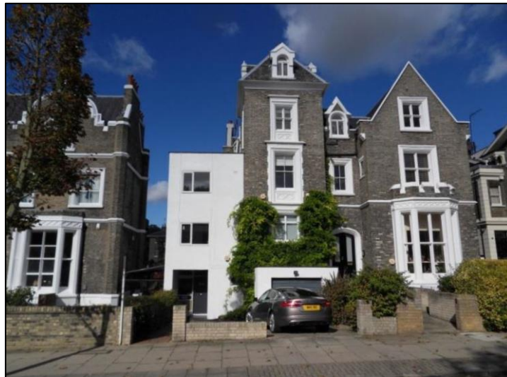
Photo 5: South elevation prior to the redevelopment (Gemini Building & Design Consultancy)
