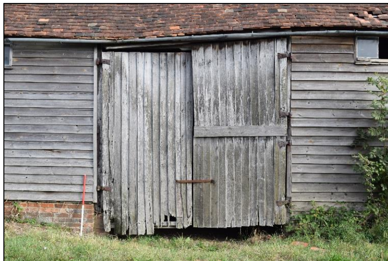
Photo 8: Exterior of the cart doors on the south elevation
