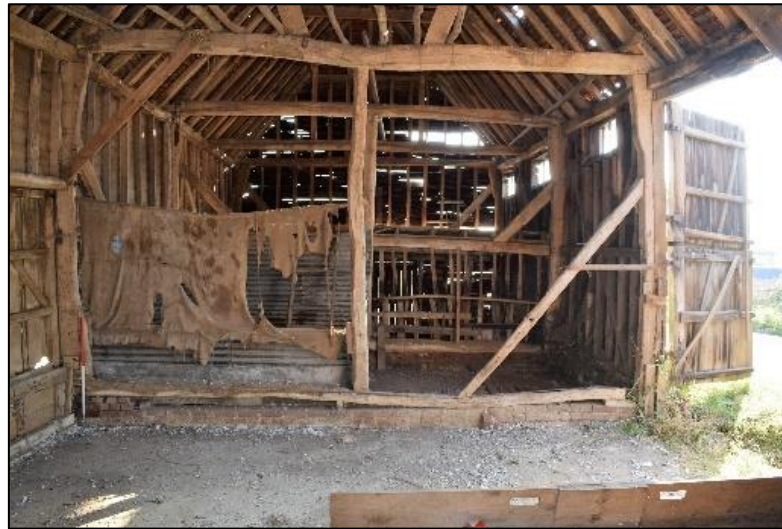
Photo 14: View of the eastern bays of the barn
