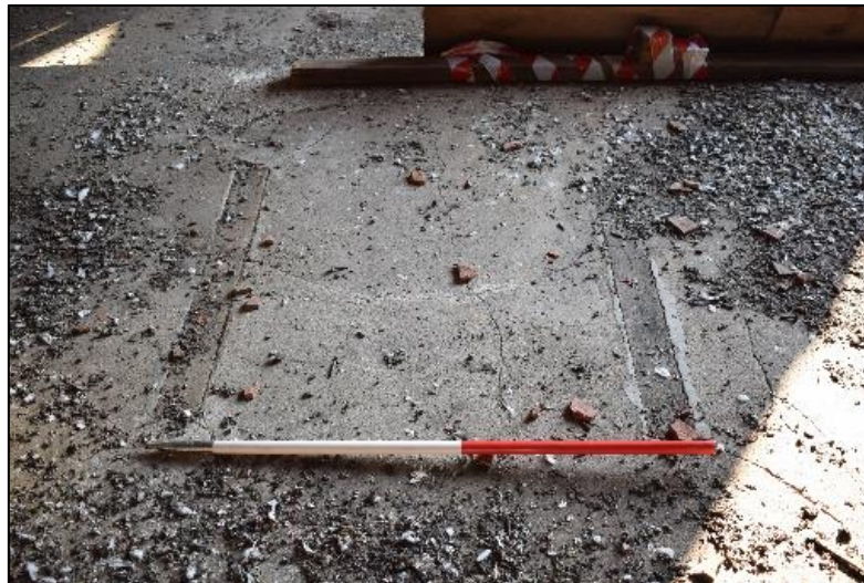
Photo 13: Timber in the floor of the western bay
