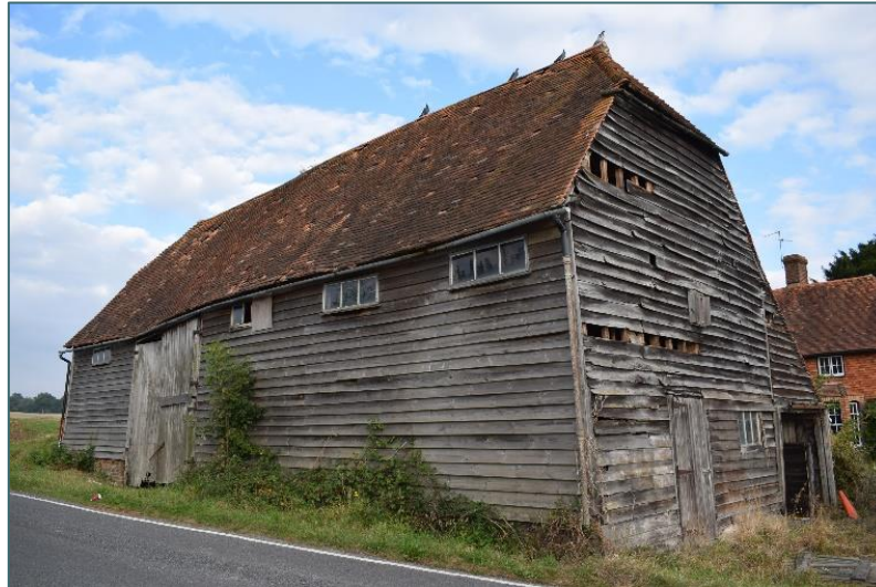
Photo 7: The south and east elevations of the barn (scale 1m)
