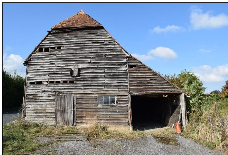
Photo 9: The eastern elevation of the barn
