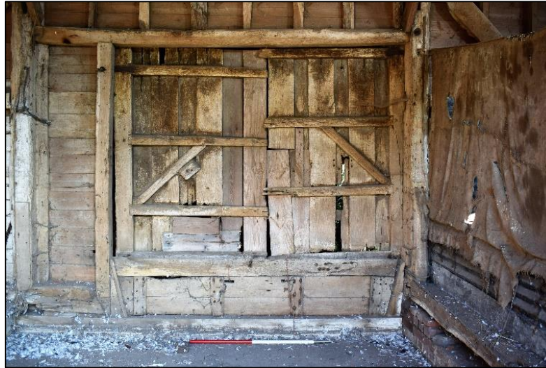
Photo 12: Winnowing door and leap at the north end of the threshing floor
