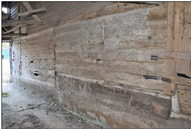
Photo 17: Area of original weatherboarding (centre) within the catslide extension
