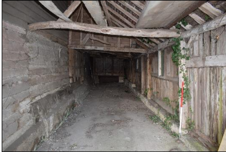
Photo 16: The extension beneath the catslide roof
