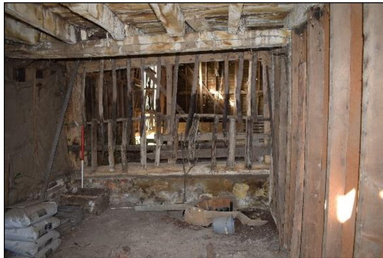
Photo 15: Ragstone foundations at the eastern end of the barn
