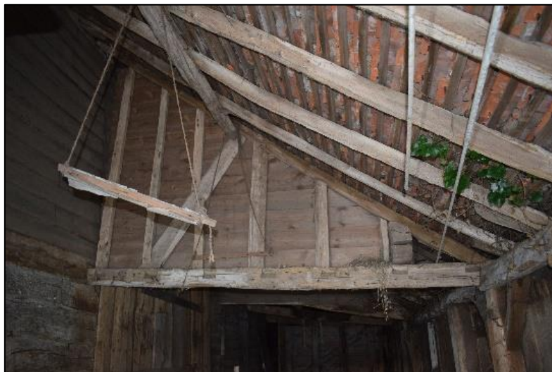
Photo 19: Re-used timber in the catslide extension
