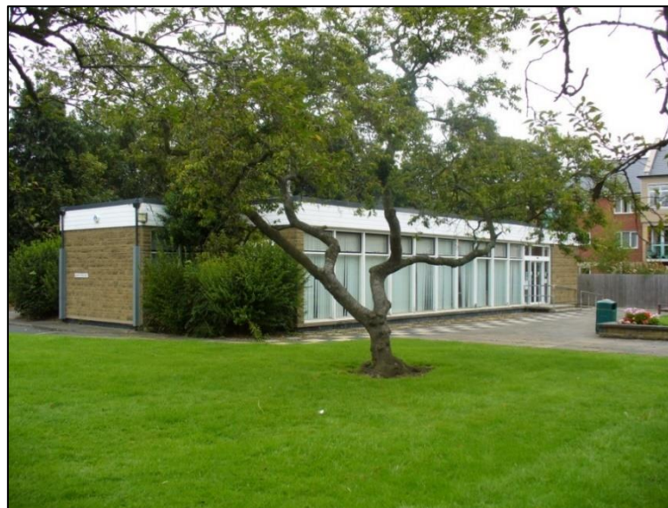
Plate 2. Showing Existing Library Building. Looking NW from Thornhill Rd
