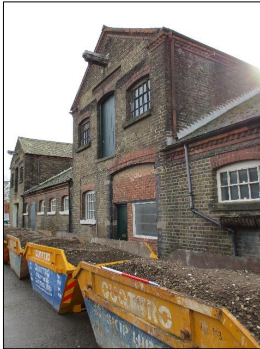
Photo 4: North-west gable from the north-west
