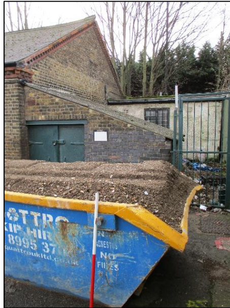
Photo 6: Extensions on the north-west elevation
