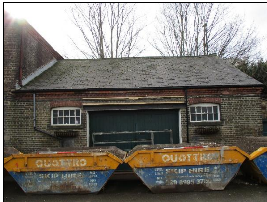
Photo 5: North-west end from the north-east
