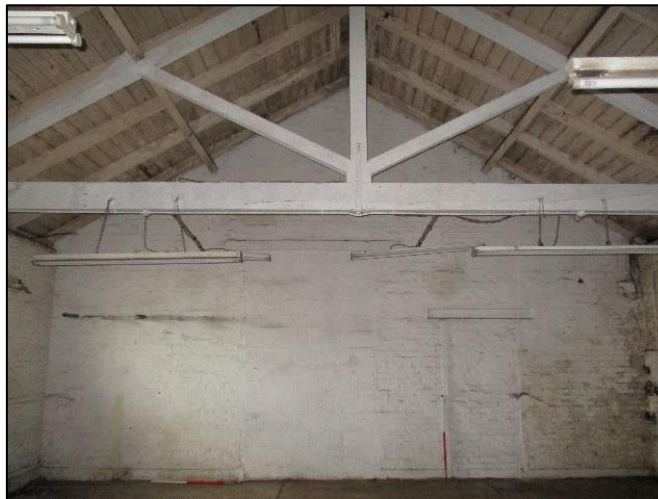
Photo 9: Blocked doorways in the north-west end of the building
