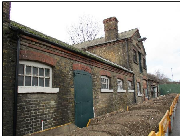
Photo 3: North-east elevation from the south-east
