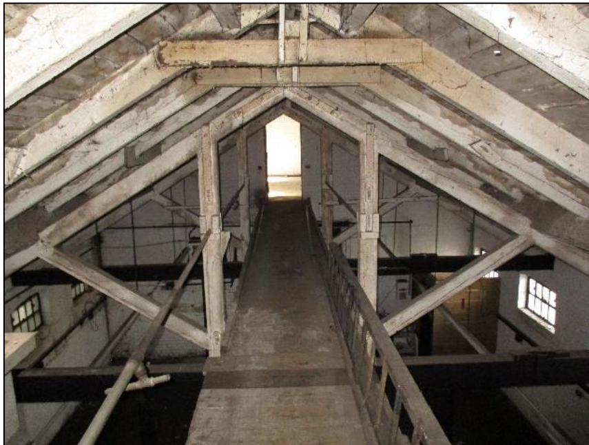
Photo 15: View along with first-floor walkway, from the south-east
