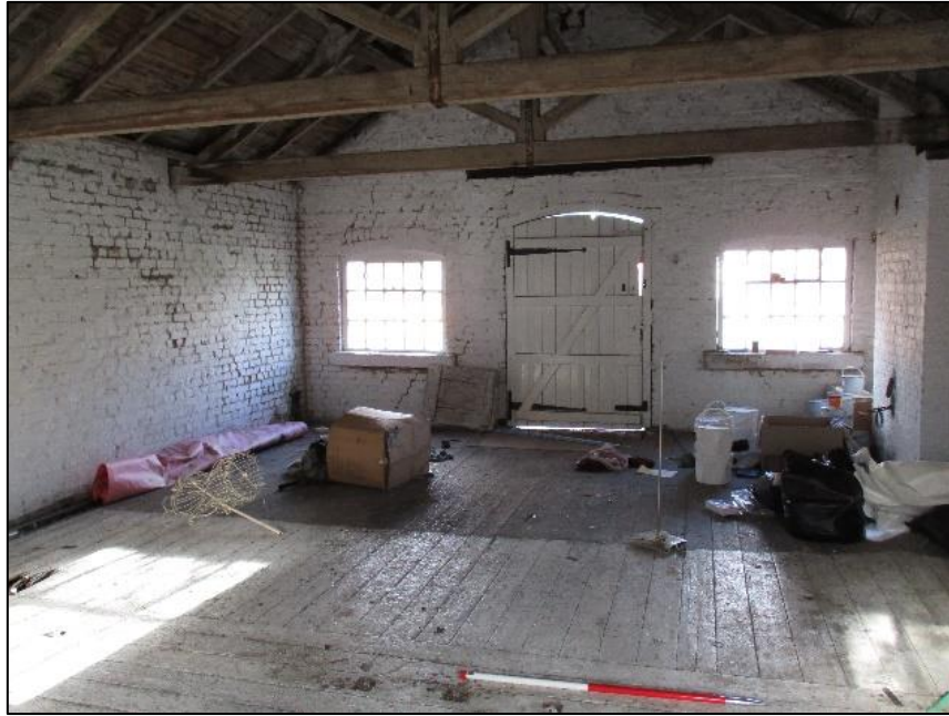
Photo 14: First floor roof structure and floor boards in the third bay
