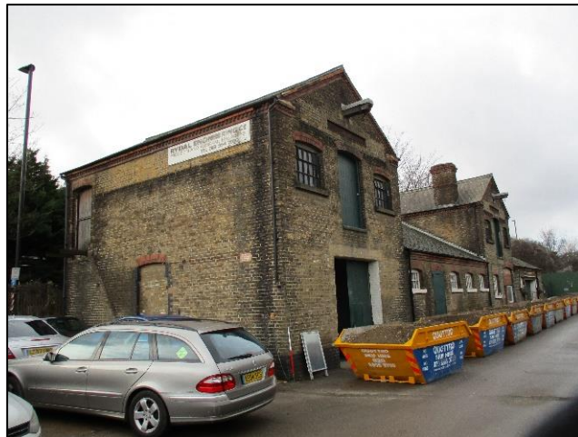
Photo 1: The former stable block from the south-east
