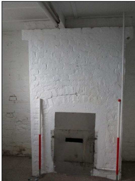
Photo 11: Chimney & fireplace in ground floor central bay
