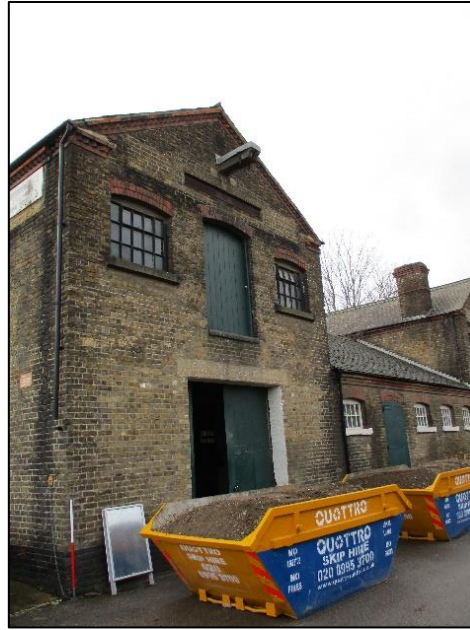
Photo 2: South-east gable end of the north-east elevation
