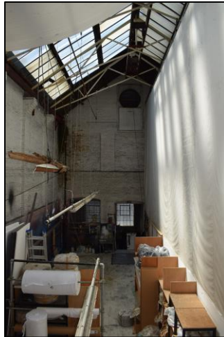
Photo 9: The first-floor space from the north-west
