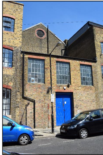
Photo 3: The rear (west) elevation from the north-west
