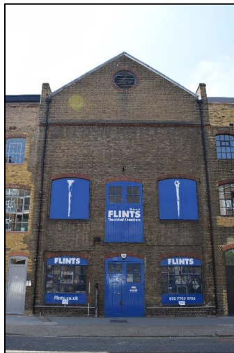
Photo 2: Front (east) elevation from the north-east (scale 2m)
