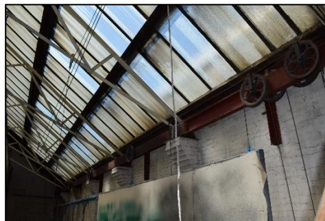
Photo 10: Surviving winch and pulley system runner frame & pulleys
