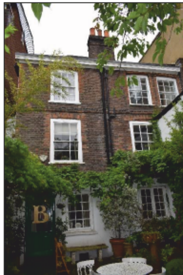
Photo 2: The rear elevation from the garden
