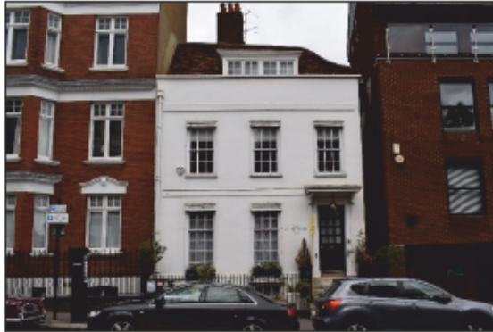
Photo 1: The front elevation from Highgate High Street, looking north
