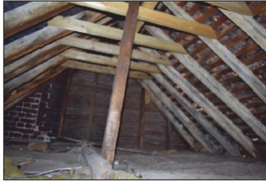
Photo 12: Part of the roof structure
