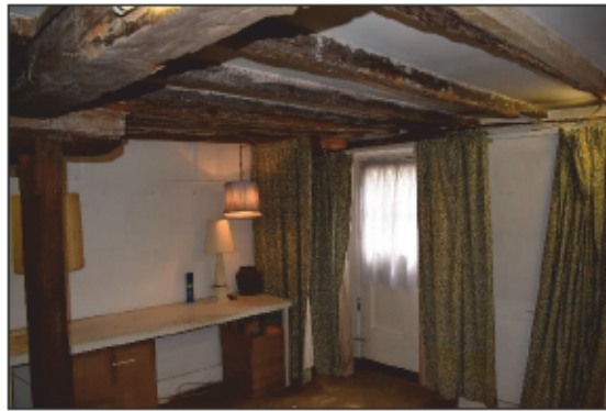
Photo 13: Ground floor timbers visible in the basement
