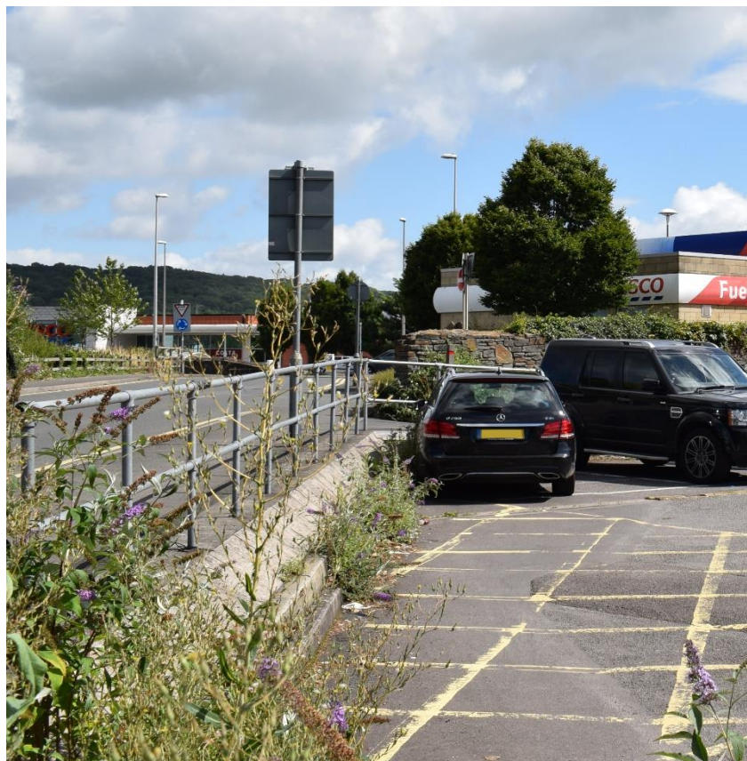
Photo. 7. Looking north into north-east corner of site, showing terraced construction of existing car park
