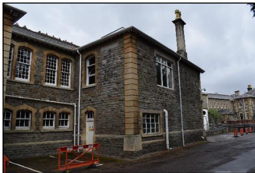
Photo 3: Inserted windows in part of the north elevation (former foul linen dept.), from the north-east
