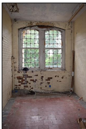
Photo 12: Quarry tile floor and blocked doorway (left) in one of the northern side rooms, looking north
