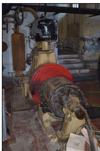
Photo 17: One of the c. 1960s steam engines in the basement powerhouse
