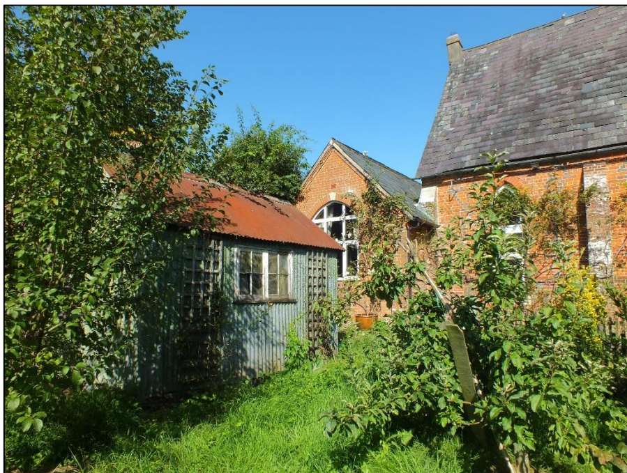
Photo 3: Corrugated iron shed in eastern half of the site
