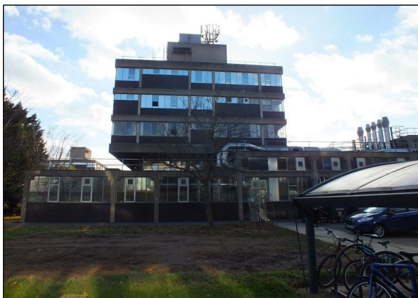
Photo 14. View of Tower A
