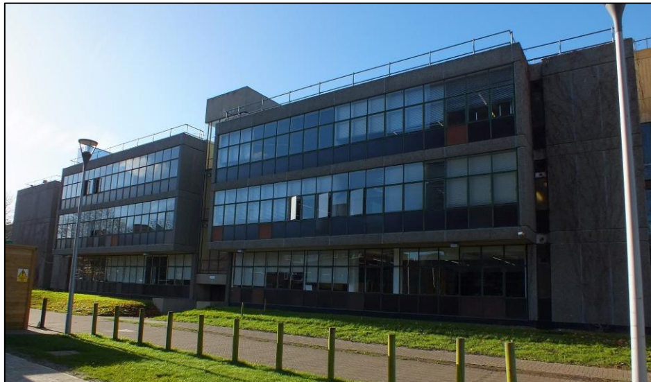
Photo 3. Southern part of CLB Eastern elevation
