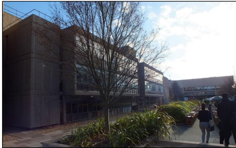
Photo 15. View of the CLB with Howell Building to the rear (shown on right)
