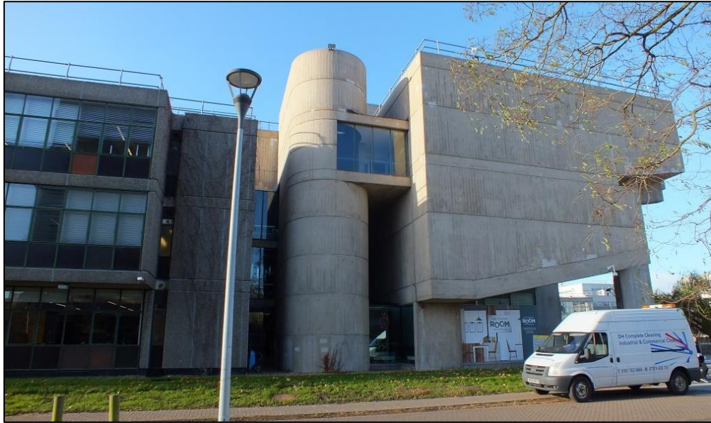
Photo 2. Northern part of CLB- eastern elevation
