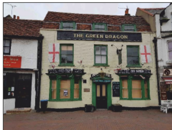
Photo 1. Showing front elevation, including modern door and signage
