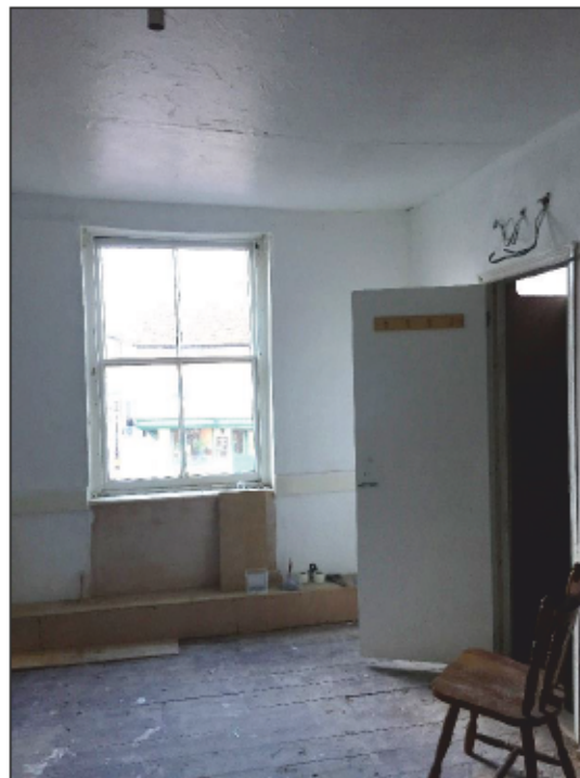
Photo 4. Showing new doorway in Room 6. Looking East
