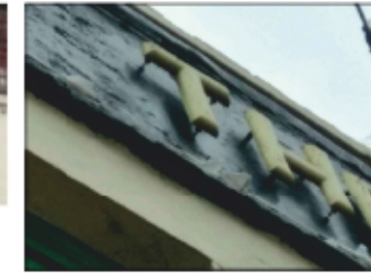
Gold leaf wood letter fixed to 18mm ply with metal dowel
