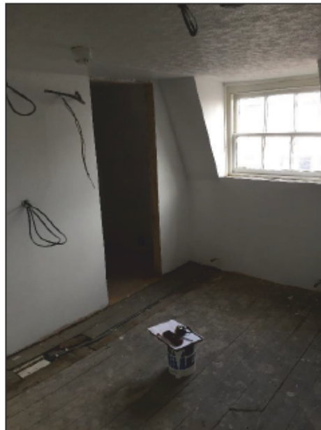
Photo 5. Showing new doorway in Room 1
