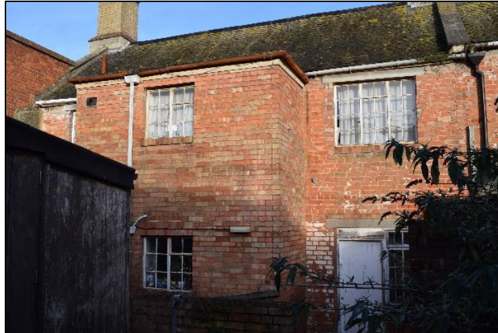
Photo 2: The rear (west facing) elevation from the rear yard
