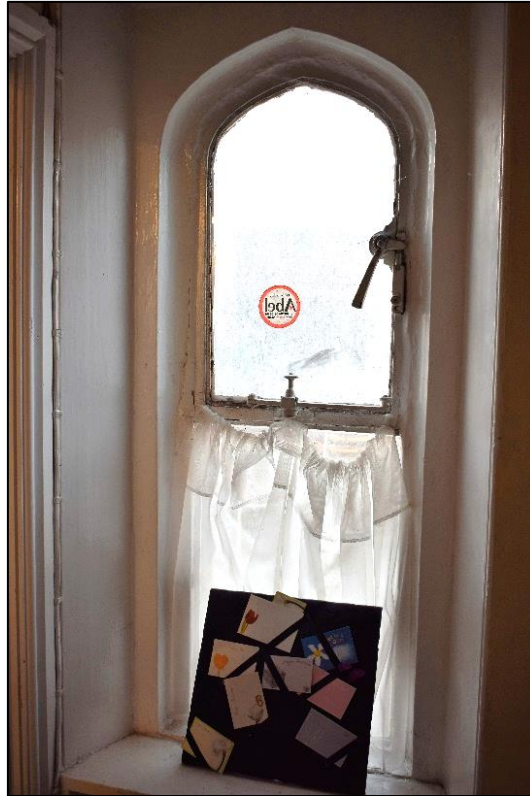
Photo 5: Original window furniture on the ground floor
