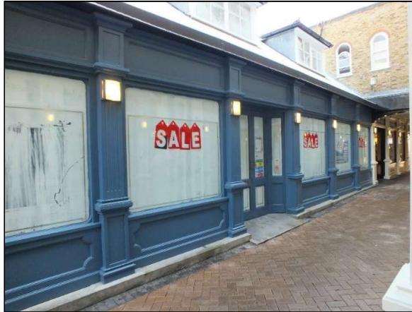
Photo 4: Shopfront on southern facade, looking north-east
