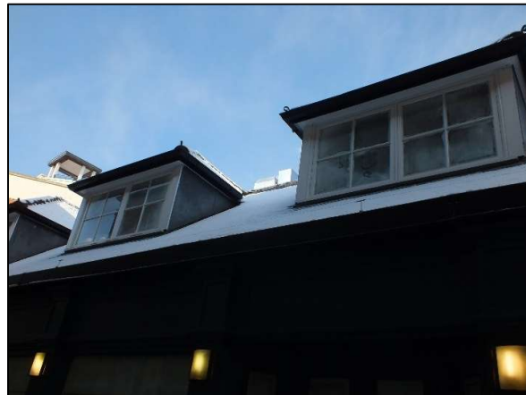
Photo 3: Dormer windows and view towards newly installed ventilation flue, looking north-west
