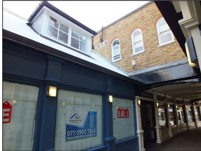
Photo 6: Rear of Unit 1, former Griffin Hotel, looking north-east
