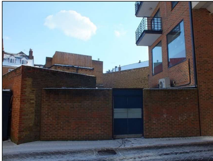
Photo 5: View towards site from Wadbrook Street, looking south-east
