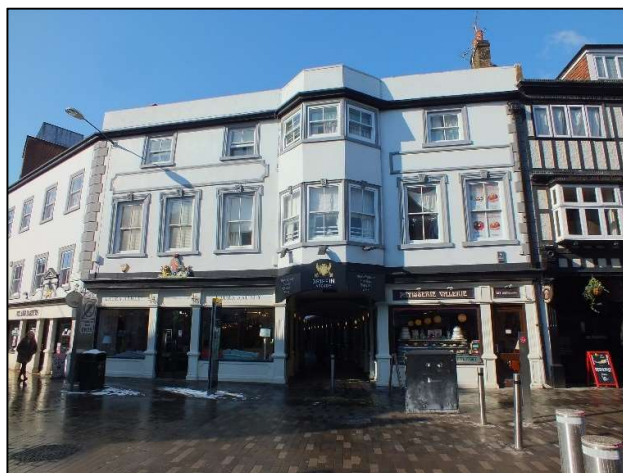
Photo 8: Street frontage of former Griffin Hotel, looking west
