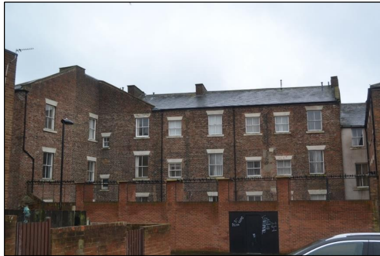
Photo 8. Looking south at the rear elevation of Liberty Court
