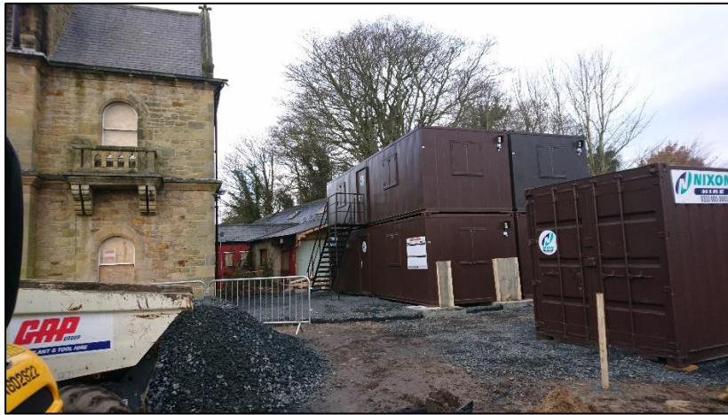
Photograph 10. Looking west at temporary construction works (2018)
