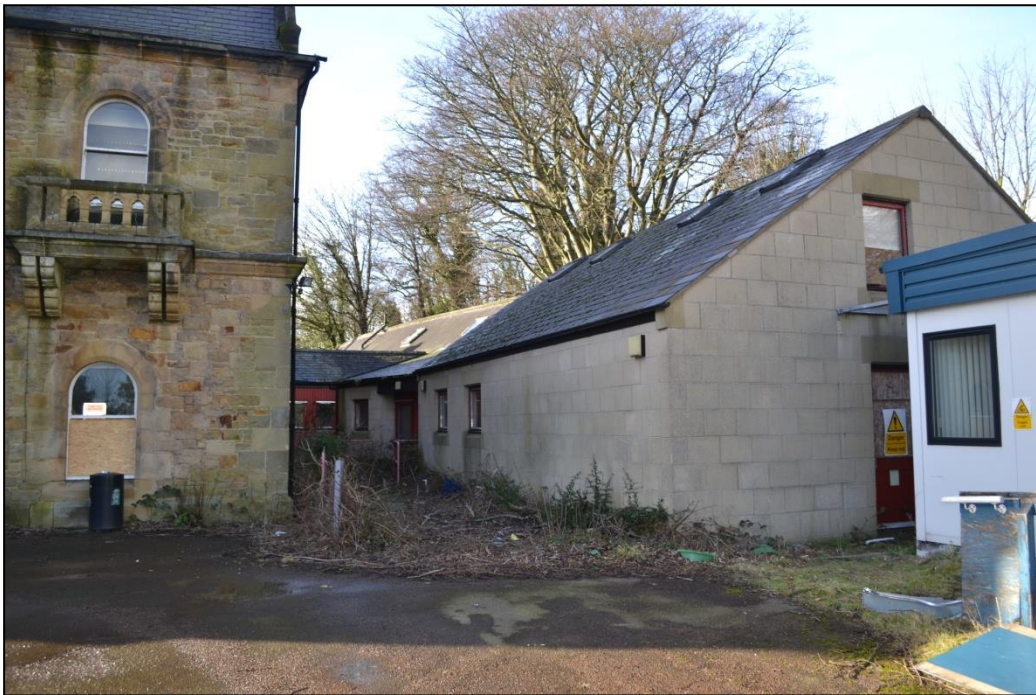
Photograph 6: Looking at District Council Era Extension at East Front (2016)
