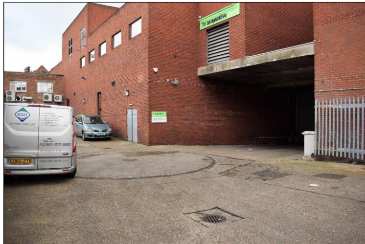
Photo 4: View into the application site, showing service covers and elevation change
