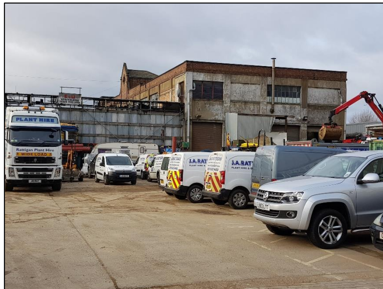
Photo 6: View of the buildings on the interior of the site from the north-east
